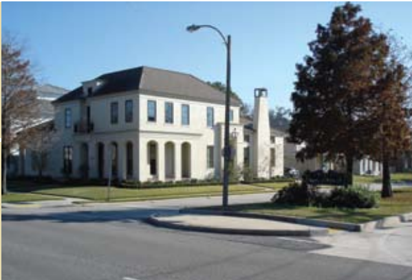
New homes in Lakeview following Hurricane Katrina.
